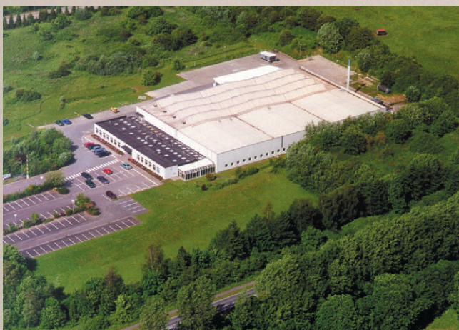
Obr.3 Danfoss Silicon Power v Schlesswigu, Nemecko
