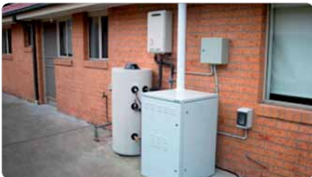
Obr. 6 TEG POWER Source-1 TEG 30 W el a TEG Power FtHeatTransfer 200W el [4]
